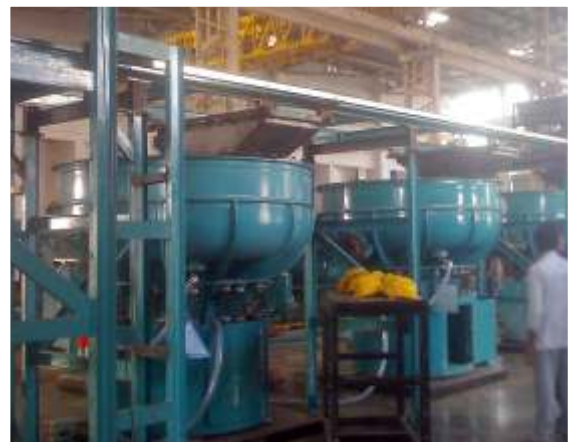
BULK LOADING SYSTEM
